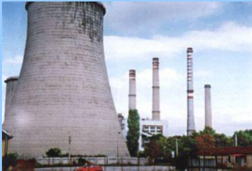
CHP Plant Sofia, Bulgaria
