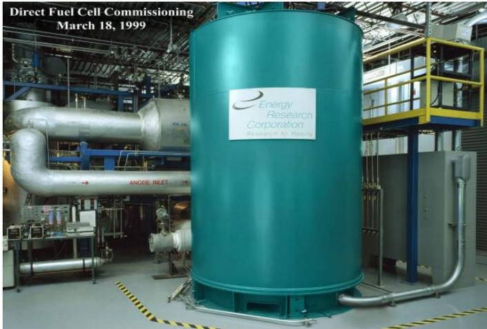
MCFC fuel cell has an electrolyte composed of carbonates that are solid at room temperature, but become liquid at 650 C, making reaction between H<sub>2</sub> and O<sub>2</sub> efficient, tolerant and “burns” CO.
