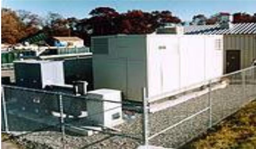
PAFC uses an electrolyte of concentrated phosphoric acid ( $\text{H}_3\text{PO}_4$ ) operating at 150-200 C and could tolerate up to 1.5% CO. It uses natural gas or propane as source of  $\text{H}_2$ .
