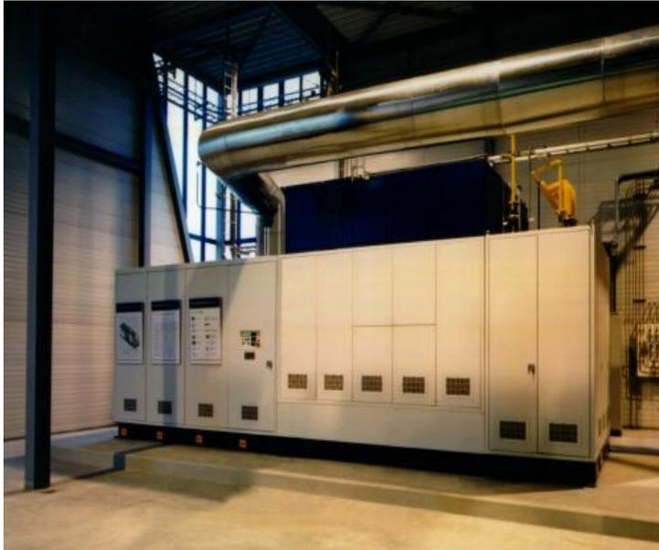
SOFC is a true solid fuel cell and contains no liquid components. Electrolyte used is a ceramic material called zirconium oxide, stabilized with yttrium oxide. To have good conductivity, it is heated to 1000 C and has efficiency of 50%. Temp could be lowered to 800 C.
