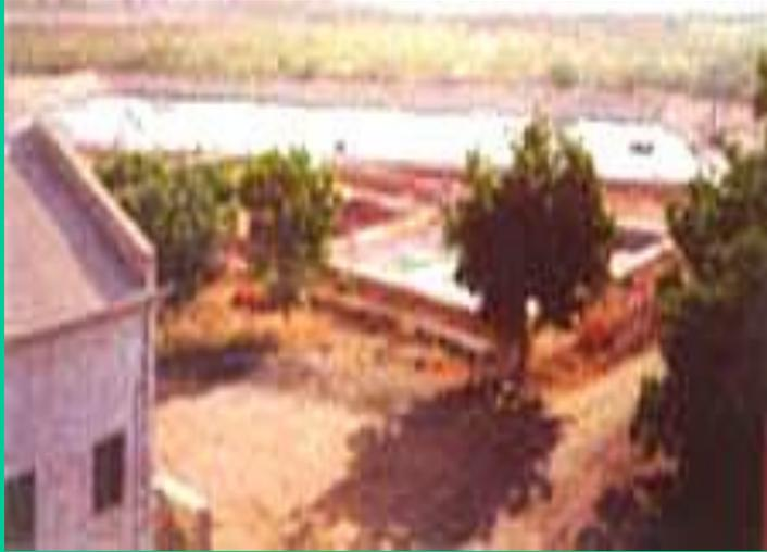
The 6000-m<sup>2</sup> in Bhuj, the first large-scale pond in industrial environment to cater to actual user demand, supplied totally about 15,000 m<sup>3</sup> (15 million liters) of hot water to the dairy at an average temperature of 75°C between September 1993 and April 1995. It is estimated that the beneficiary of the project, Kutch Dairy, can save over 935 metric tons of lignite per year if the solar pond is used to its full capacity. This translates into monetary savings of of \$19,000/yr.
