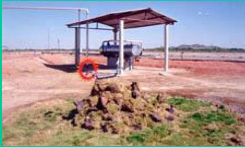
The heat extraction system consisted of brine suction and discharge diffusers, a brine pump, associated piping, controls, and instrumentation. Both the suction and the discharge diffusers were installed on the same side of the pond. Keeping in view the problem of fouling, a shell-and-tube type heat exchanger was chosen. Brine was on the tube side, which was made of cupro-nickel. The pond is capable of delivering 80,000 liters of hot water daily, at 70 degrees C or above.
