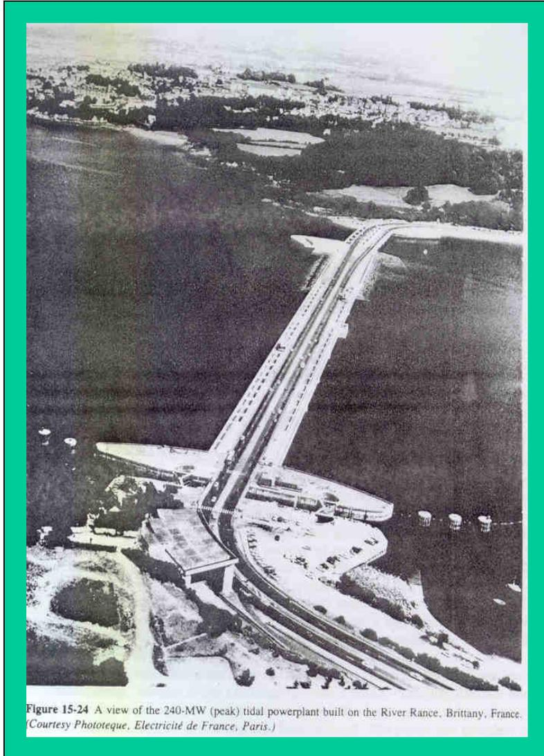
Figure 15-24 A view of the 240-MW (peak) tidal powerplant built on the River Rance, Brittany, France. (Courtesy Phototeque, Electricité de France, Paris.)
