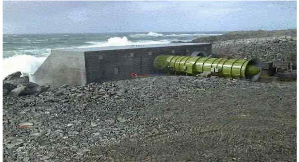
LIMPET generates 500 kW, uses inverter drive for high turbine efficiency, 60-year service life, connected to UK's national grid with a 15-year PPA, costs 1 million pounds, and provides power to 400 island homes. Overall efficiency of up to 40% under ideal oscillating flow with the use of intelligent controller for varying rotor resistances.
